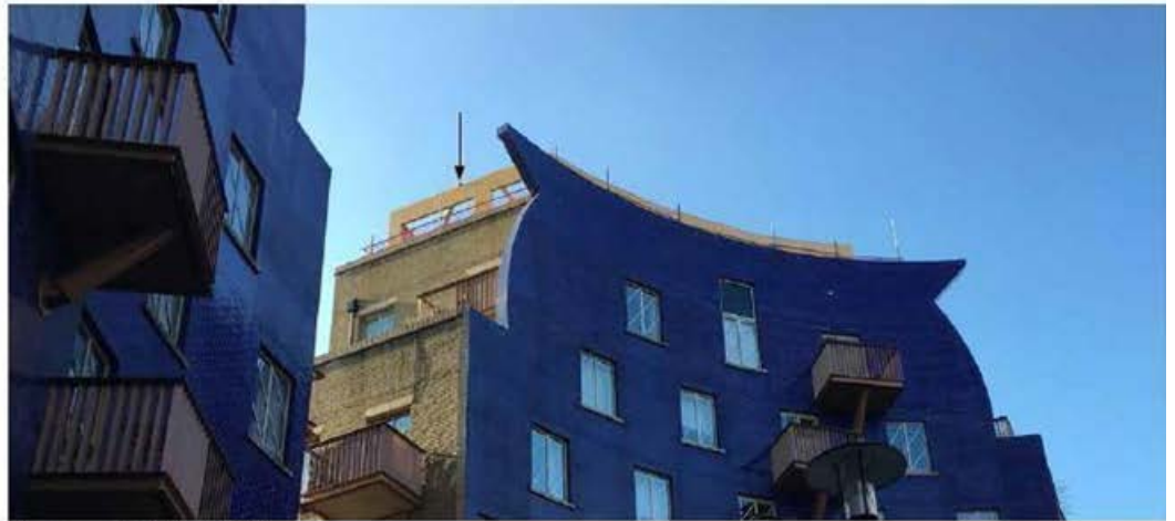
Site progress under NMA 15/AP/0060
