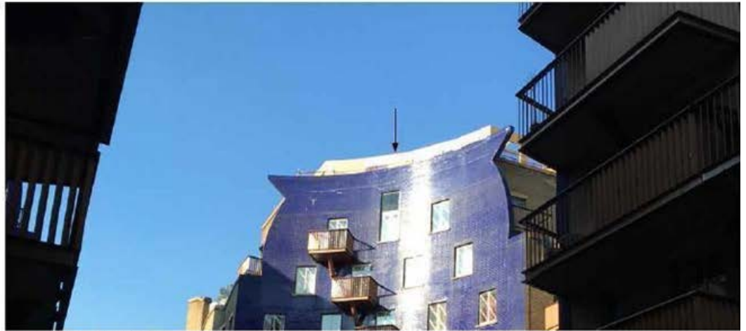
Site progress under NMA 15/AP/0060
